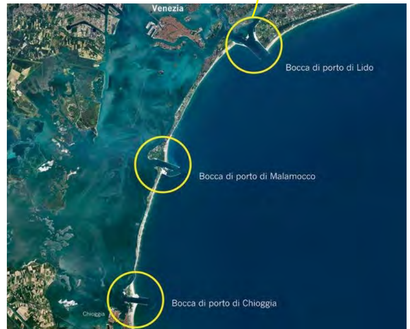
MOSE flood walls under construction to protect Venice, Italy from high tide flooding and rising sea levels.
