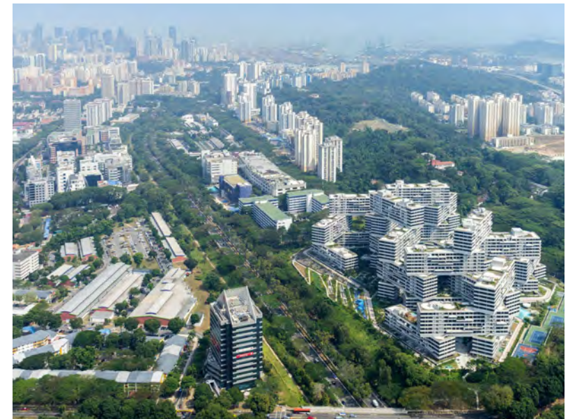
Top: Hospitals in Singapore include interior green space to promote physical health and mental well-being for patients, visitors and staff (Pictured Khoo Teck Puat Hospital). Bottom: Green corridors and natural areas built into the urban fabric.
